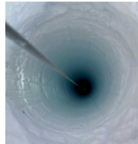
Drilling, installation of antennas at a depth of over 100 m
