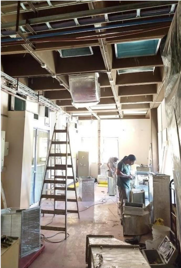
35m 2 added to cleanroom
