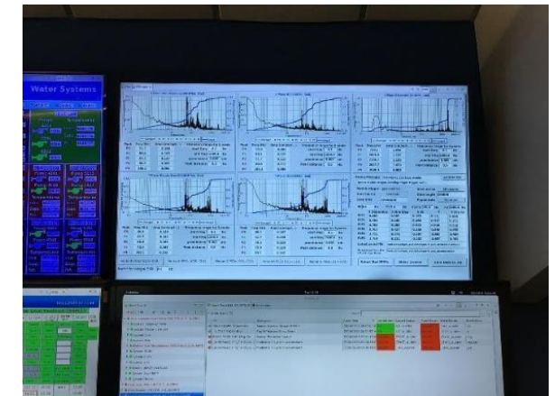
NSLS-II Control Room
