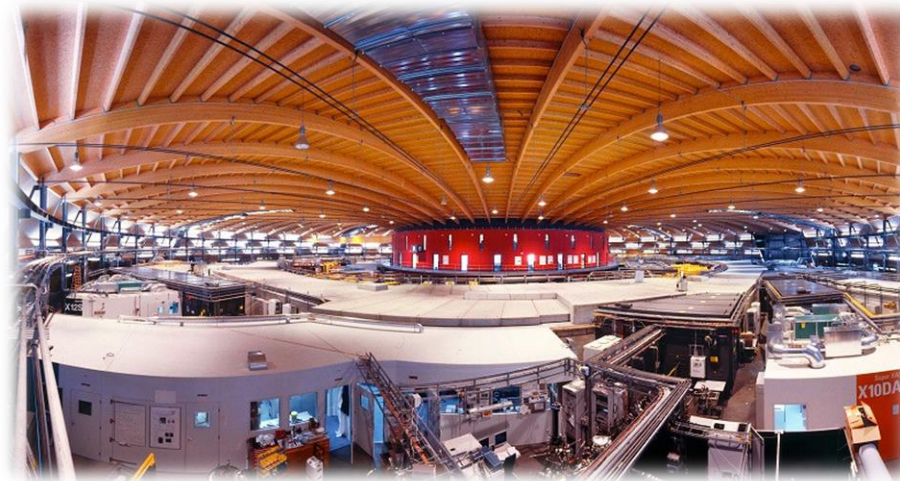
Figure 1 - Interior view of the Swiss Light Source (SLS) In user operation since 2001.
