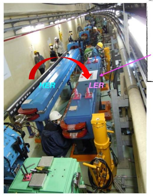
All 100 4 m long dipole magnets have been successfully installed in the low energy ring (LER)!
