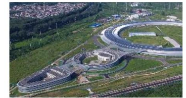
Nov. 3, 2023 Civil Construction for ancillary buildings completed
