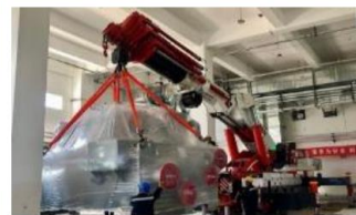
Apr. 13, 2021 Utility installation in NO.2 Hall commenced
