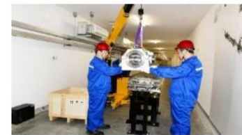
June 28, 2021 HEPS Installs First Piece of Accelerator Equipment in Linac Tunnel.
