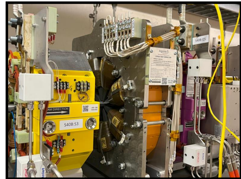
Slow and fast corrector magnet based on APS-U design
