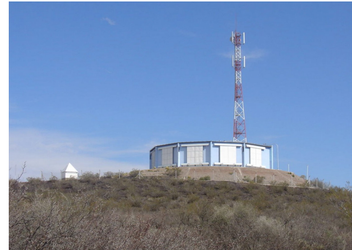
Fluorescence Detector (FD) 27 telescopes, 15% duty cycle
